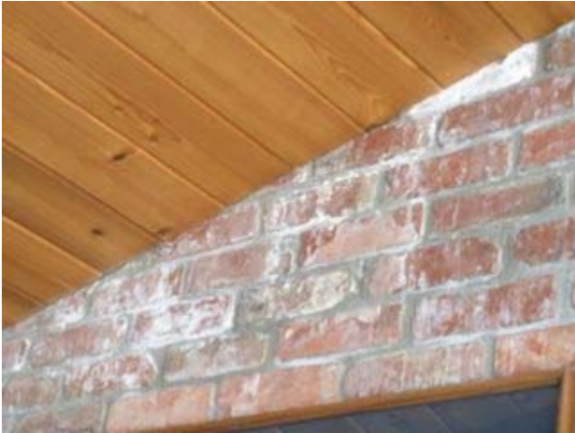
Photo 17 LR efflorescence
