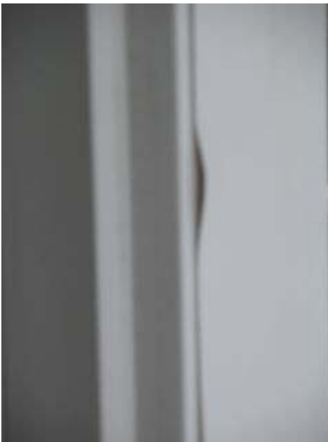
Photo 14 Warped vinyl covering
