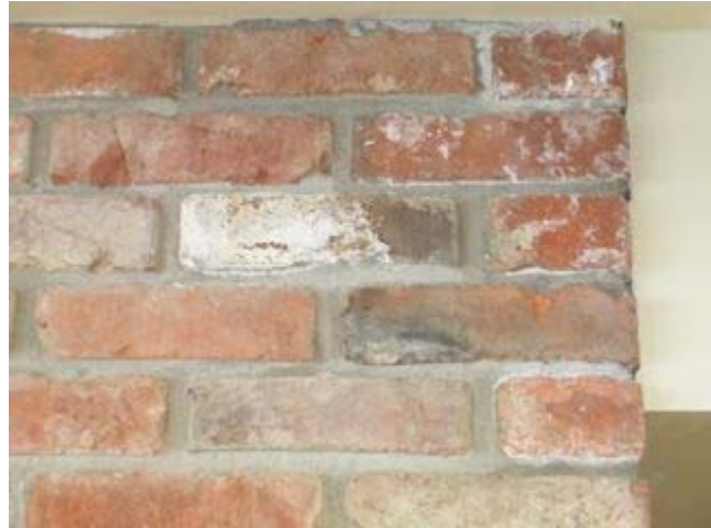
Photo 18 Kitchen efflorescence
